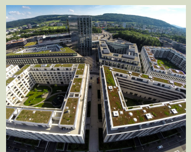
The revitalisation of roofs in the 20th century.
