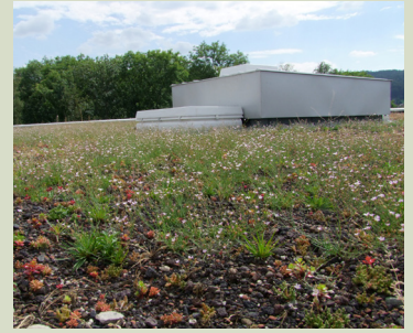
Extensive green roofs are a quasi-natural form of vegetation.
