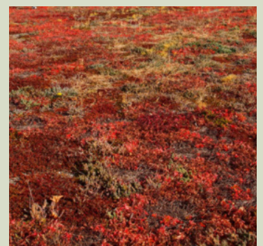
The sedums set the roof alight with their bright colours, characteristic of the autumn season.
