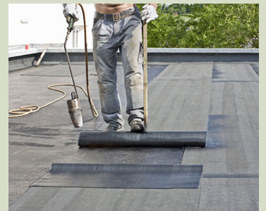
Renovation of the waterproofing of a flat roof.
