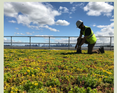
Maintenance of green roofs.
